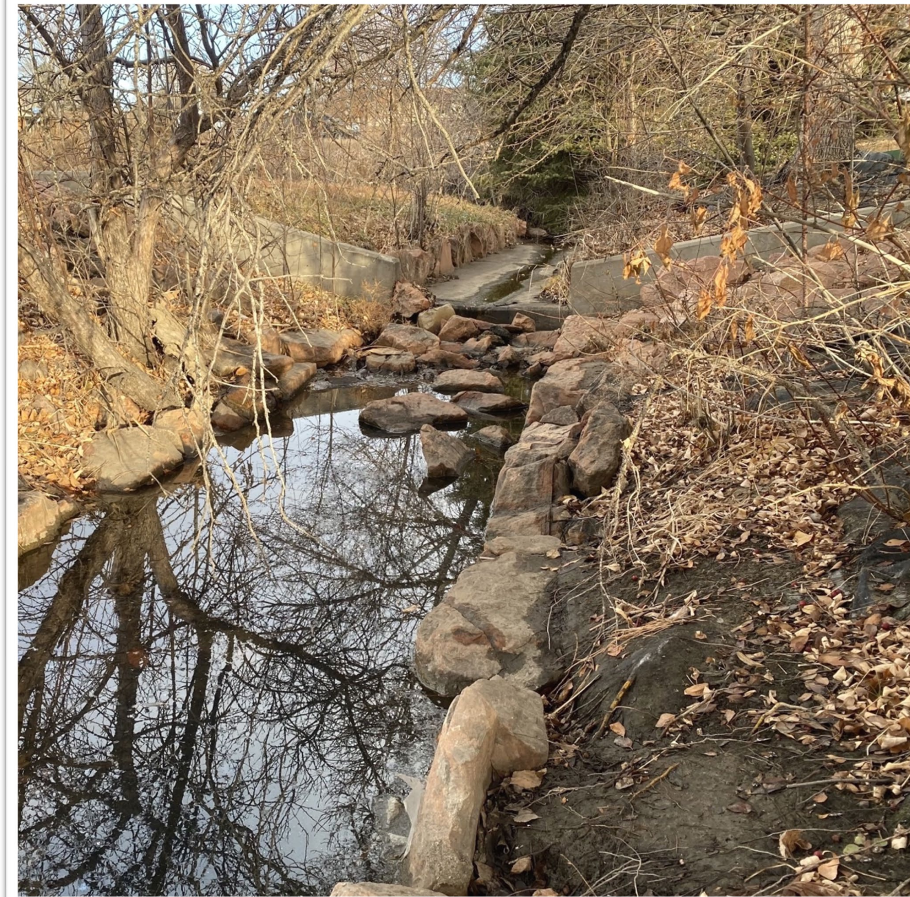
Nissen Reservoir at Main Street
